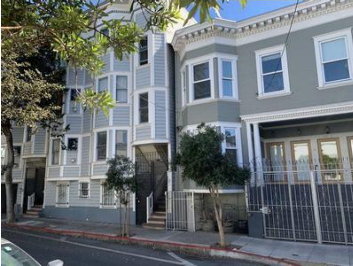
Residential buildings southwest of site
